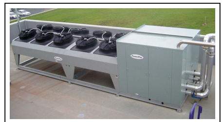
Air Cooled chiller installation
